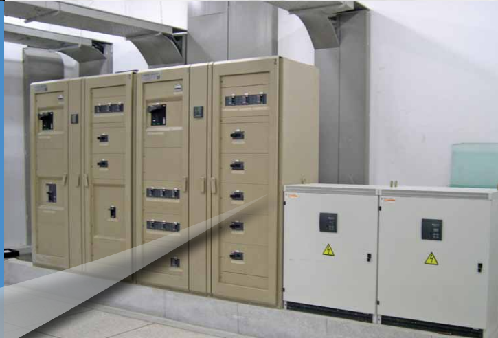
Armoire générale BT PRISMA / LT general electric cupboard PRISMA
