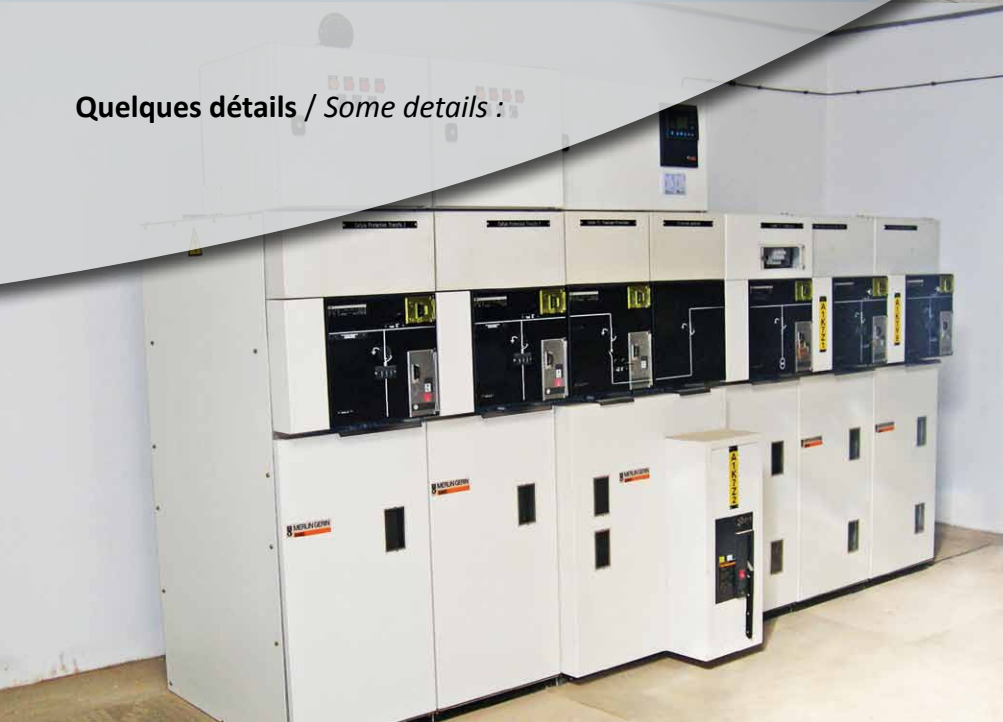
Poste de transformation 2x1000 KVA / Post of transformation 2x1000 KVA
